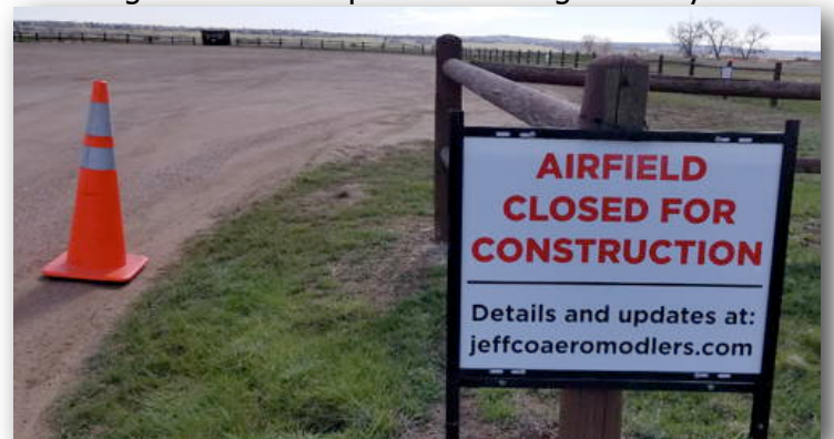
The LRPC reported the new runway project was underway and the field was closed for construction
