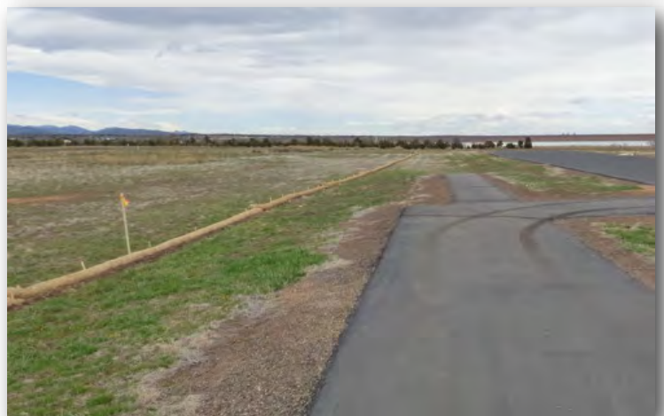
Erosion control log preparation and installation.
