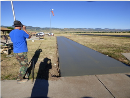
The new taxiway is poured and ready for finishing.
